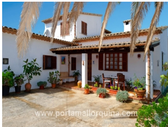
Patio and covered terrace with seating
